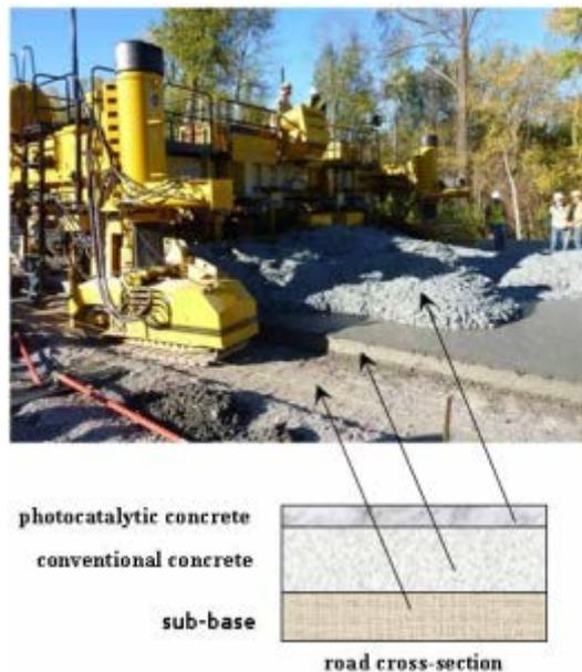
Fig.2. Application of photocatalytic – technology on Route 141 in Sent Louis,USA[4]
